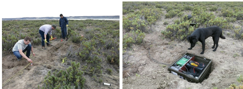
Installation of the Hugo ELF station in Colorado, USA, in May 2015
